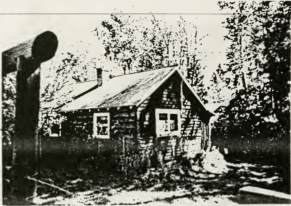
Figure 56. Structure complex #12, log house, south end.
